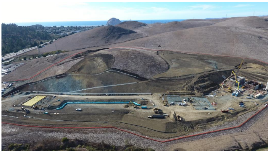
$138 Million Water Reclamation Facility (WRF) Project
